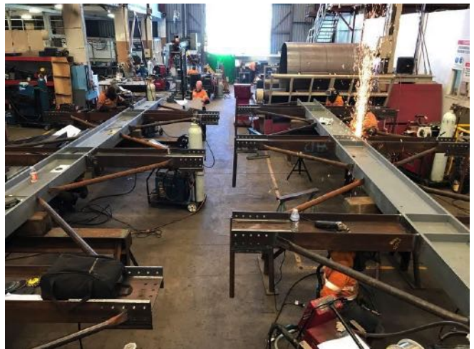
Structural columns – Novotel Christchurch
