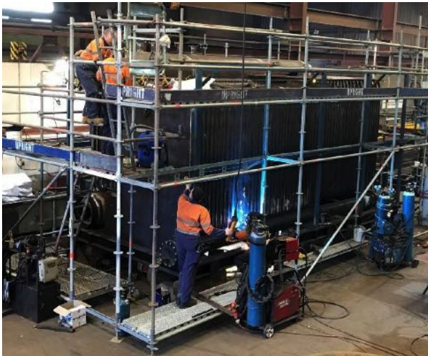
4 MW wood waste boiler under construction
