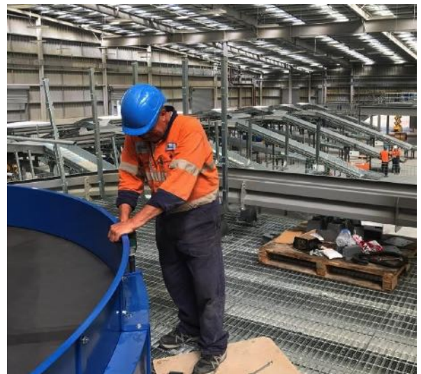
Parcel sorting plant installation
