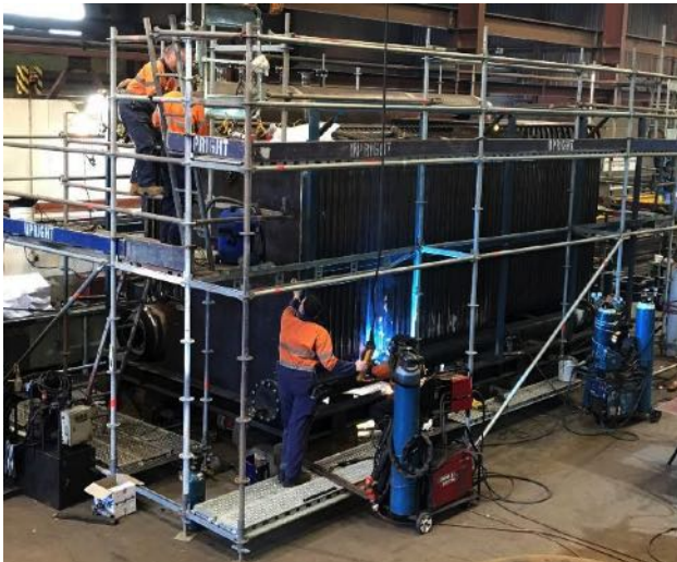
4 MW wood waste boiler under construction
