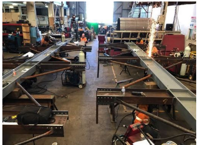
Structural columns – Novotel Christchurch
