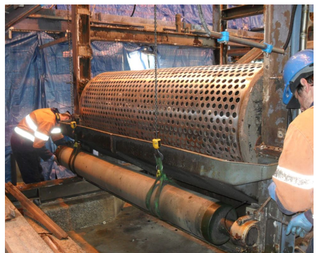
Sludge press overhaul – Waste Water Plant
