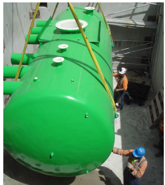
Vacuum tank installation – Prestons Road
